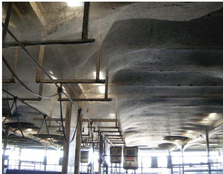
Fig. 3. Laminar webbing covering ceiling (right side of photo), grading into volumetric webbing between trolley beam hangers (left side of photo).
