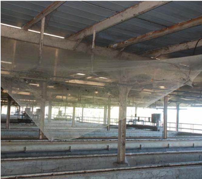
Fig. 10. Partially detached sheet of webbing (about 6.5 m across) from beneath ceiling.
