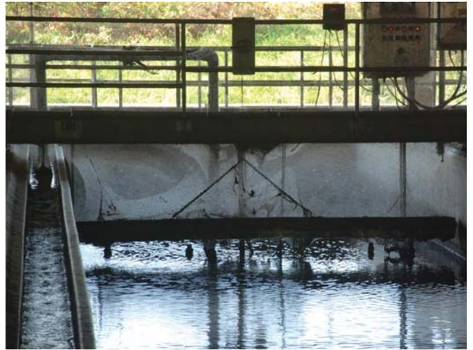
Fig. 8. Webbing beneath traveling bridge.
